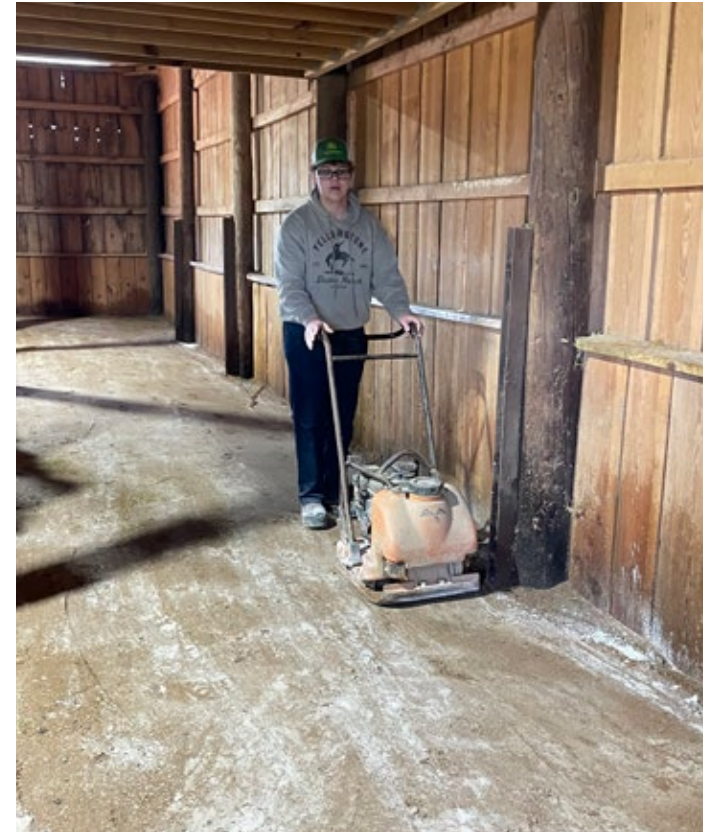
The equine center makeover was a multi-layered project that included extensive cleaning out of old shavings, tearing out the stall dividers, adding new sand and lime to the stalls and the meticulous installation of the new mats and reconstruction of the dividers.
