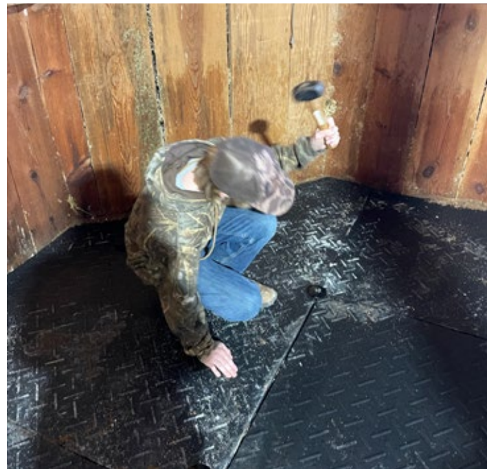
Eli Waystack, who took lead on the project, hammers in one of the stall mats.
