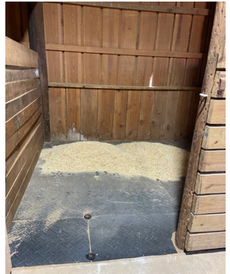
The equine center makeover was a multi-layered project that included extensive cleaning out of old shavings, tearing out the stall dividers, adding new sand and lime to the stalls and the meticulous installation of the new mats and reconstruction of the dividers.
